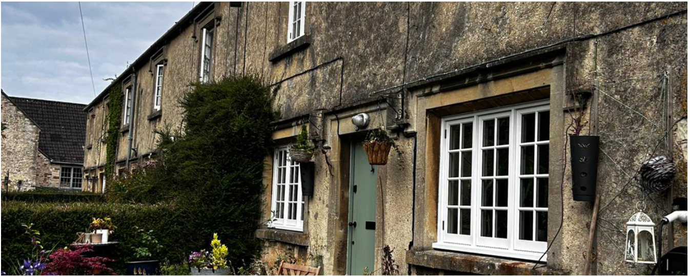
Pictured: Hand-built windows and doors at Church Street, Kilmersdon
