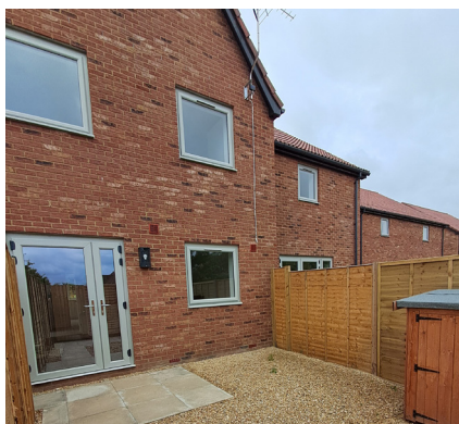
Pictured: Sheds and floor coverings provided..
