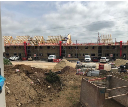
Pictured: Onsite at Sutton Benger
