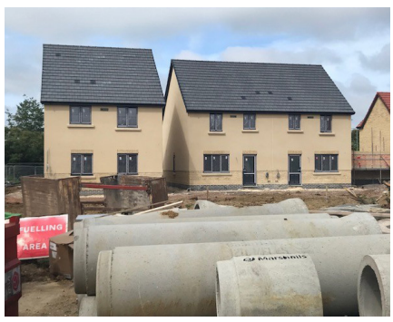
Pictured: Our new development at Garden Close, Sutton Benger nearing completion.
