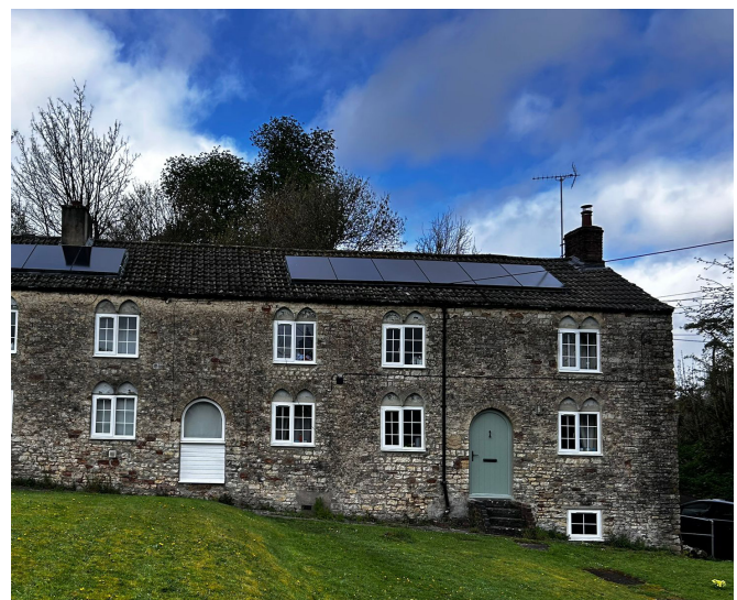
Pictured: Ammerdown Terrace - new roofs, replacement windows and Solar photovoltaic panels
