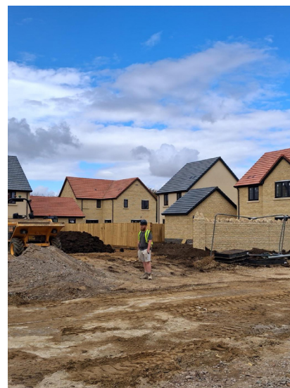
Pictured: Onsite at Hills Homes Garden Close development in Sutton Benger.
