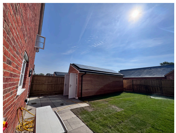
Pictured: Townsend Farmyard, Poulshot - large shed with fitted solar panels to roof.
